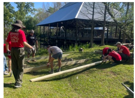
Foard Fereday leads Scout Troop 769 in Prairieville to complete his Eagle Scout project at Hilltop – a bridge across the pond overflow.
