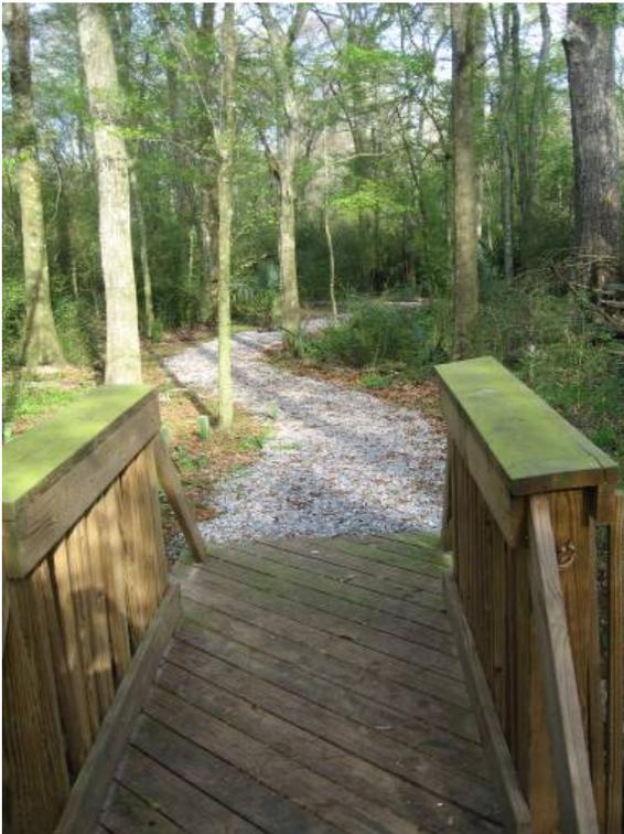
**Figure 85: After the bridge the path surface is crushed limestone.**
